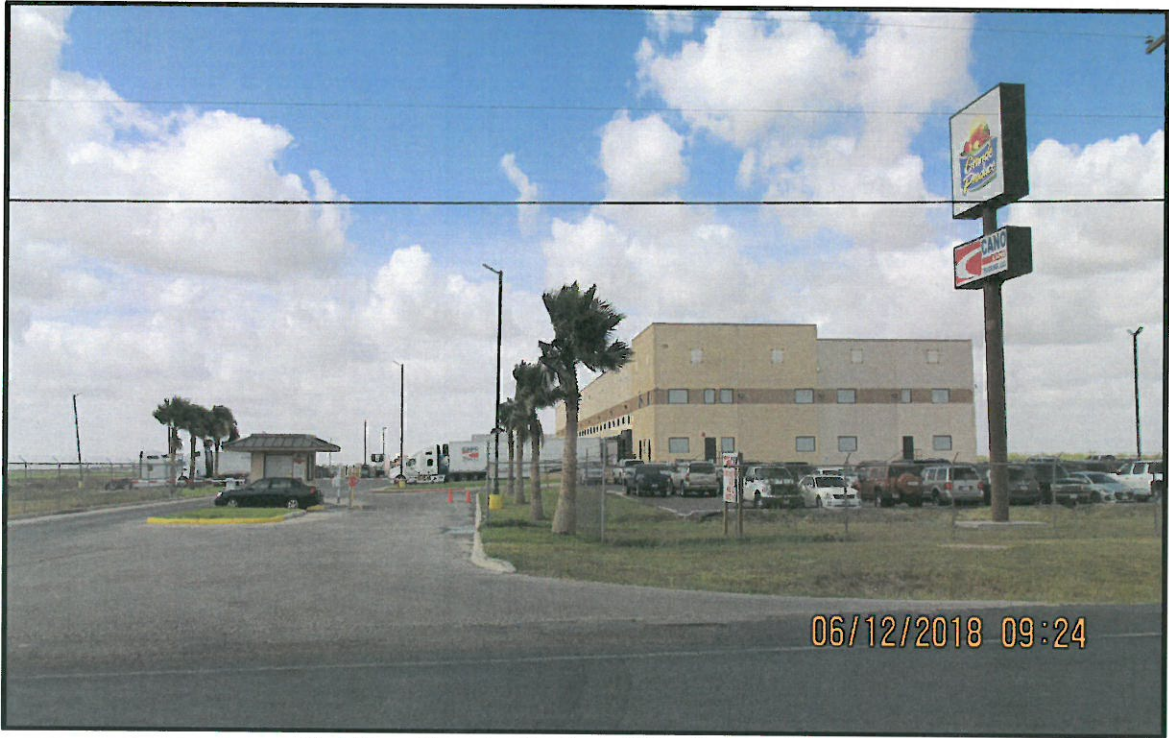
Existing Grande Produce Warehouse (West)
