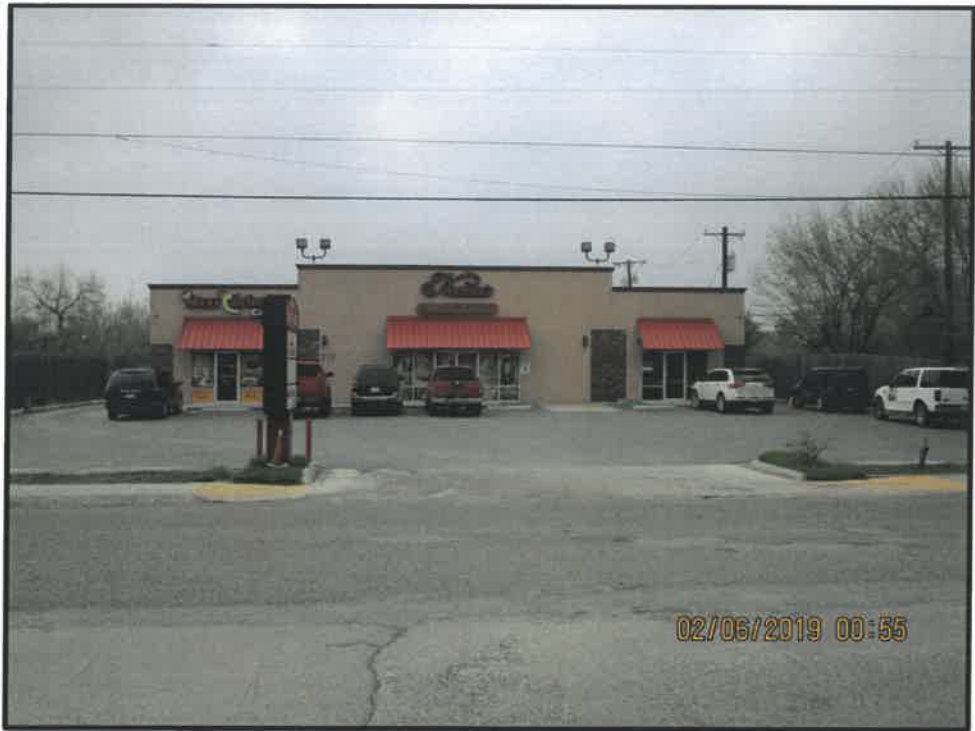
Existing commercial plaza
