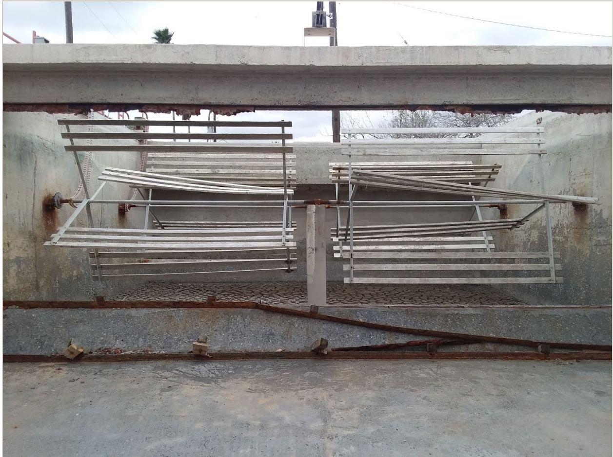
Existing Wooden-Paddle Horizontal Flocculator Background. Also visible is the steel frame of the original Flocculator Baffle Wall.
