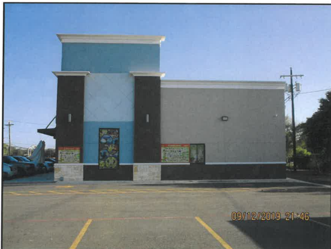
View from Second Street
