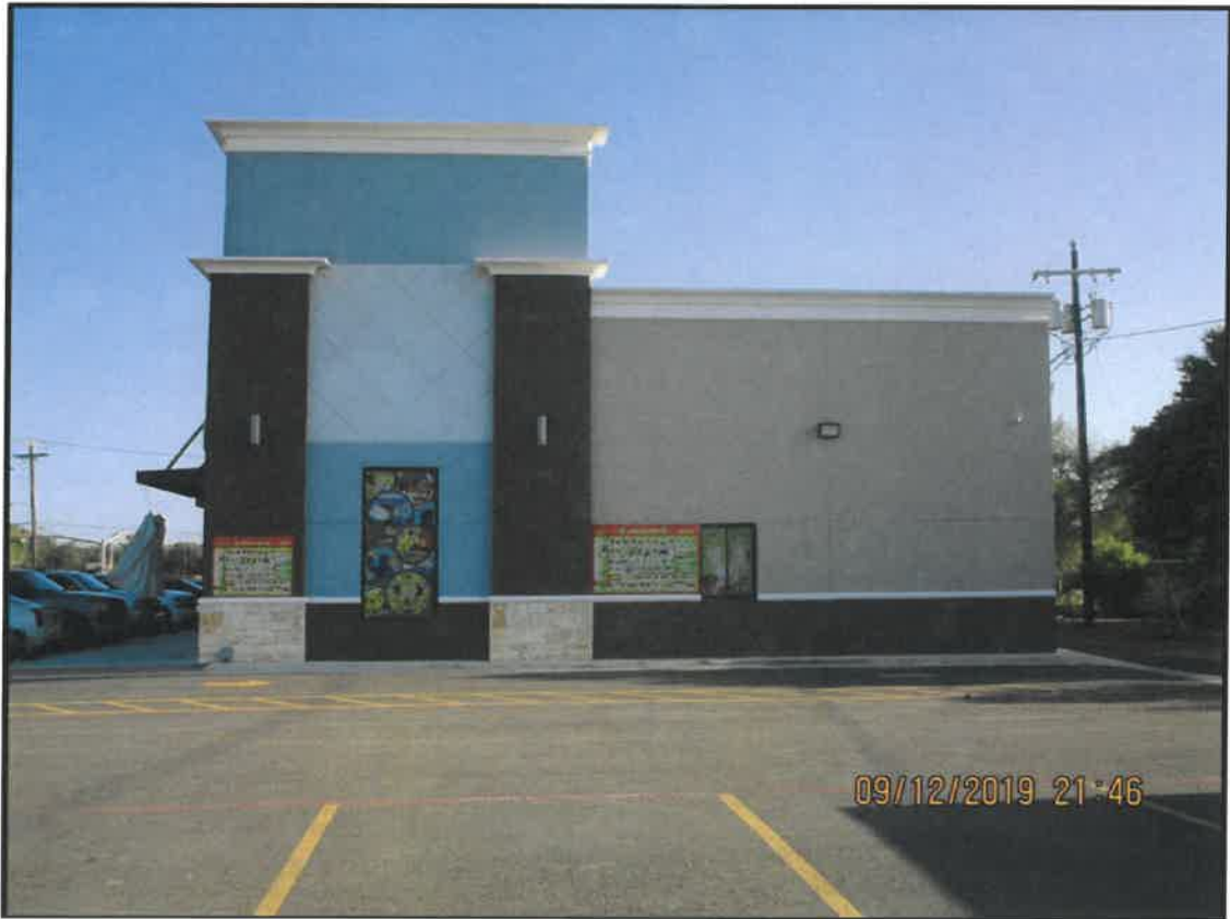
View from Second Street
