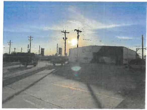
Location of Overhead Electric Line on Lot 2. Probable dedicated easement.
