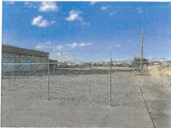
Location of Overhead Electric Line on Lot 3. Probable dedicated easement.
