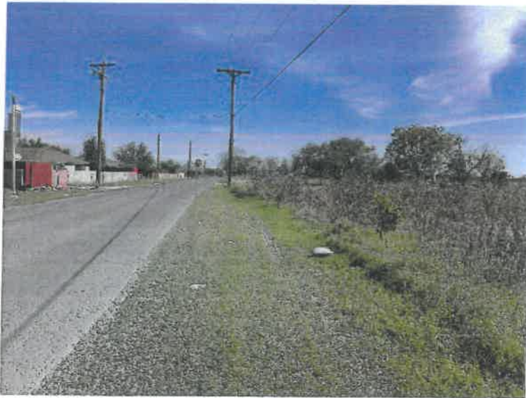
Continue with sidewalk and relocate electric poles
