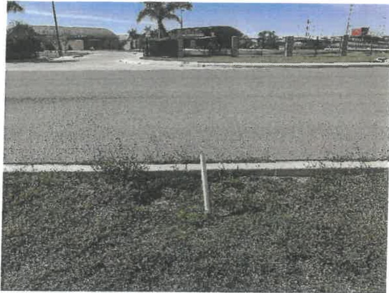
Exist. spot location not shown on plans. What is the purpose of this?
