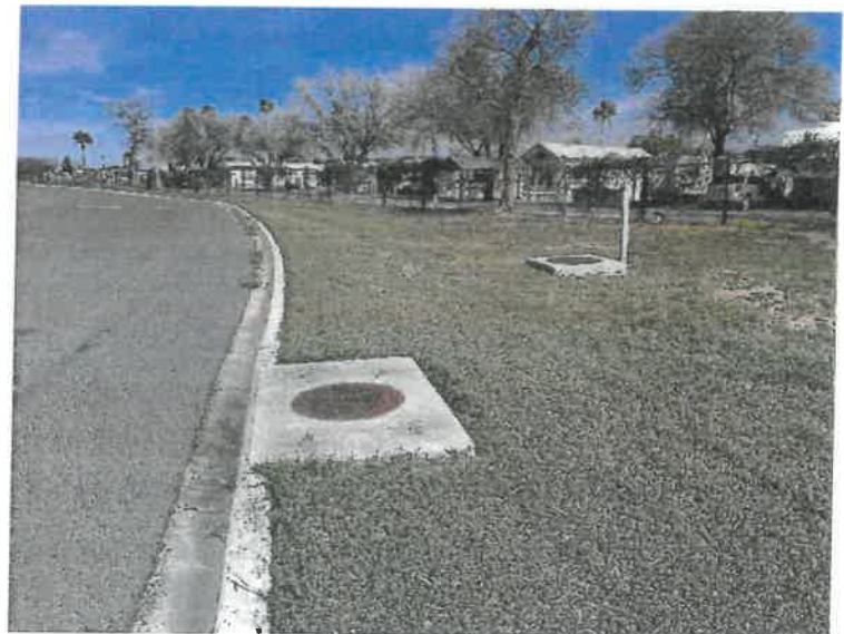
Exist. Curb Inlet. Provide information on exist. drain line
