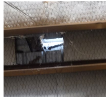
Inside of roof
