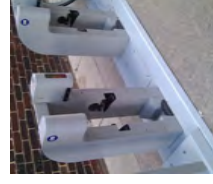
Bolted single-sided base plate
