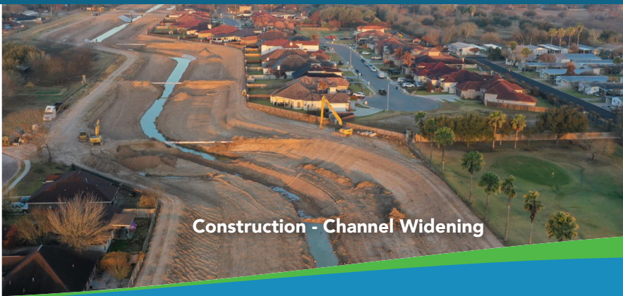
After - Expanded Channel for More Capacity
