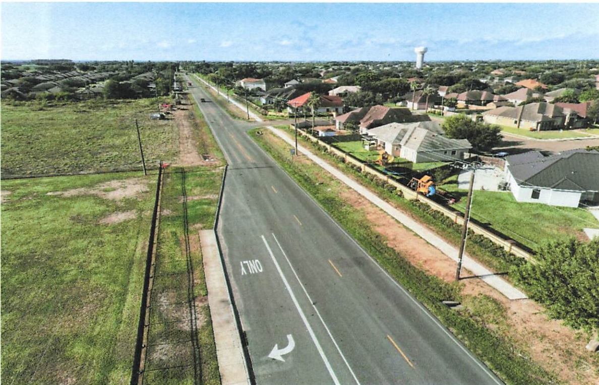
Picture No. 4. Sidewalk completed along the west side of S. Stewart Rd. south of E. Sam Houston Blvd.
