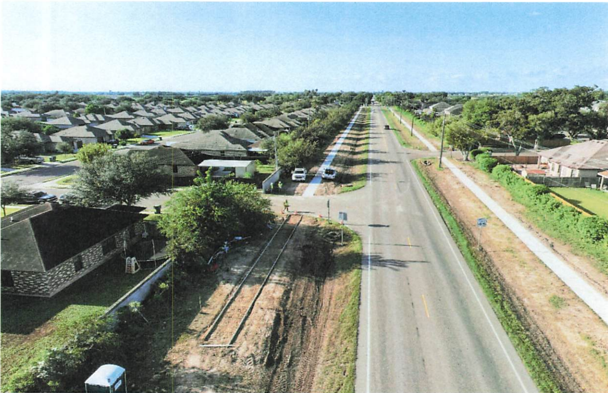
Picture No.3. Sidewalk (84 L.F.) on the east side of Stewart Rd. north of E. 13 ½ St. poured on 09/18/24.
