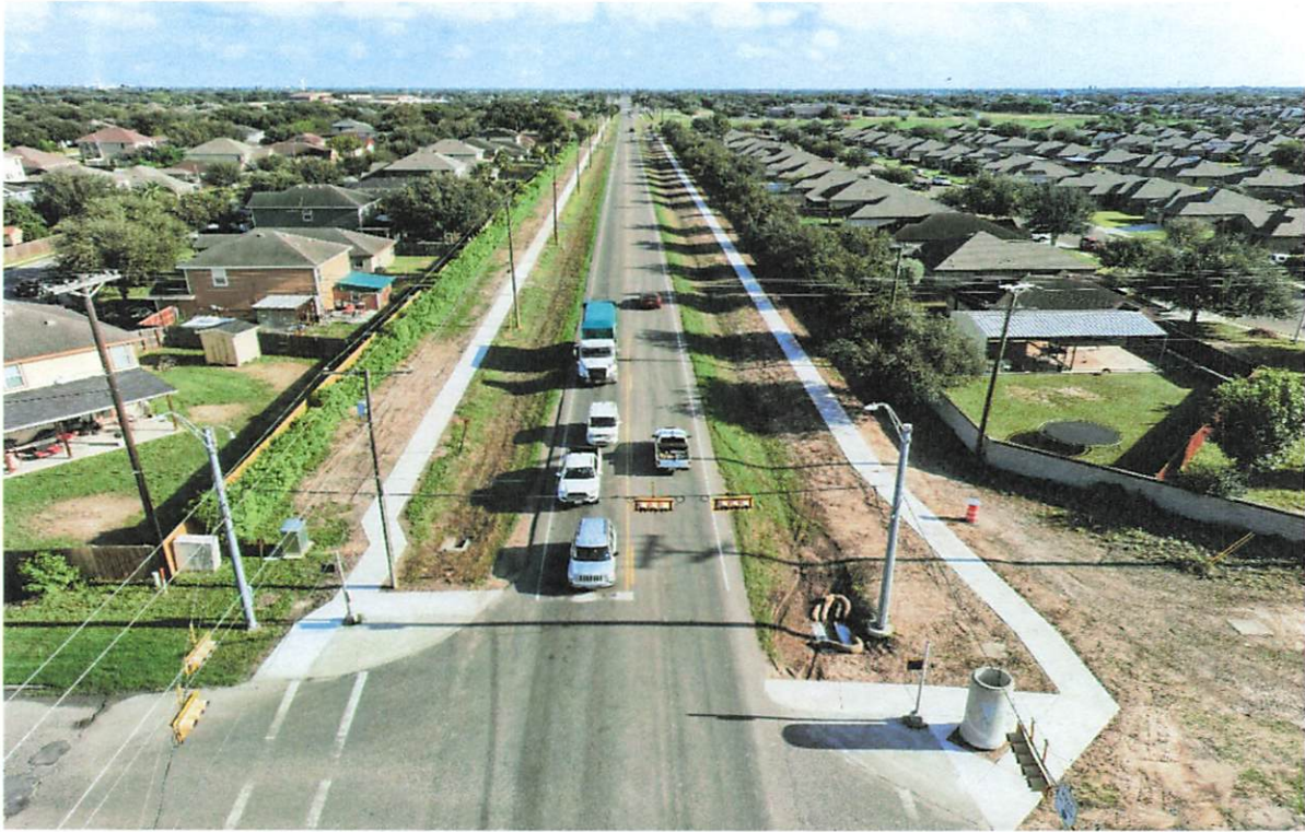
Picture No.1. Sidewalk completed along the east and west side of Stewart Rd. north of E. Ridge Rd.
