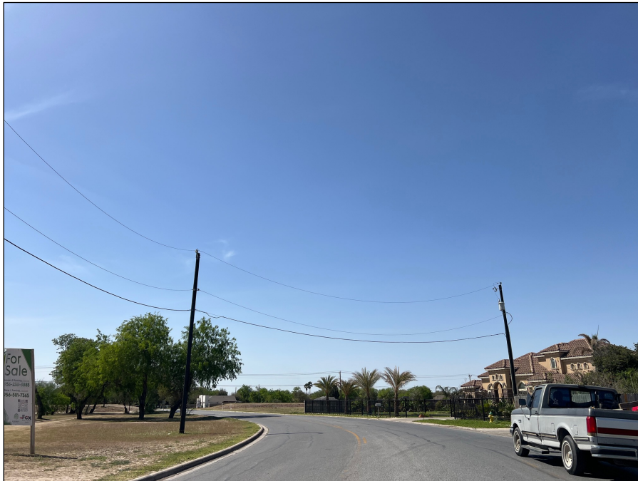
Westbound 1 st Street
