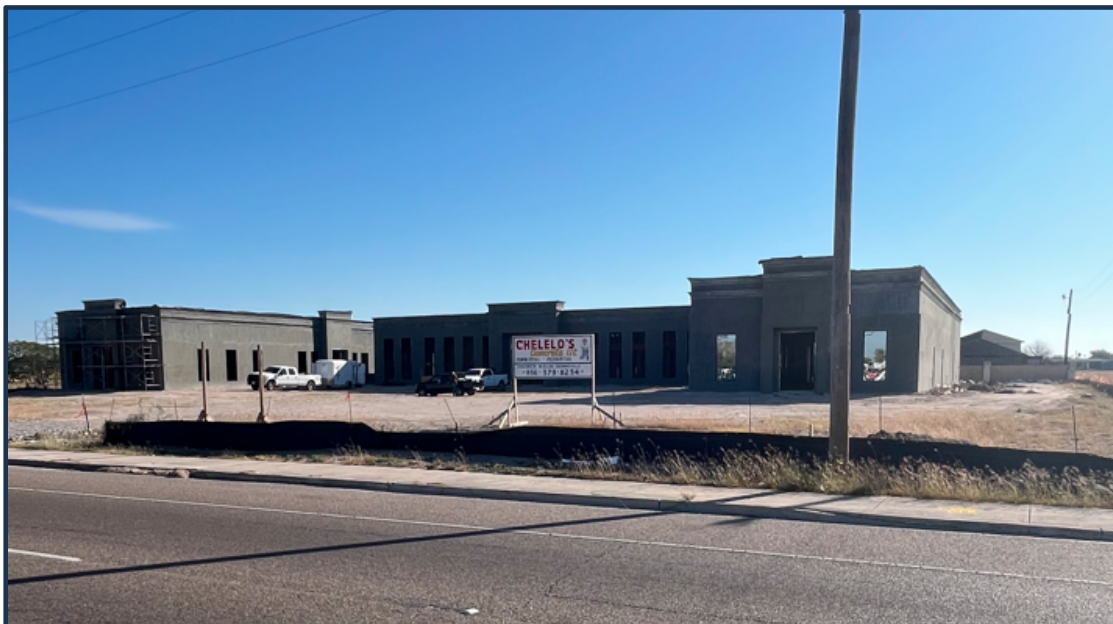
Commercial plaza under construction
